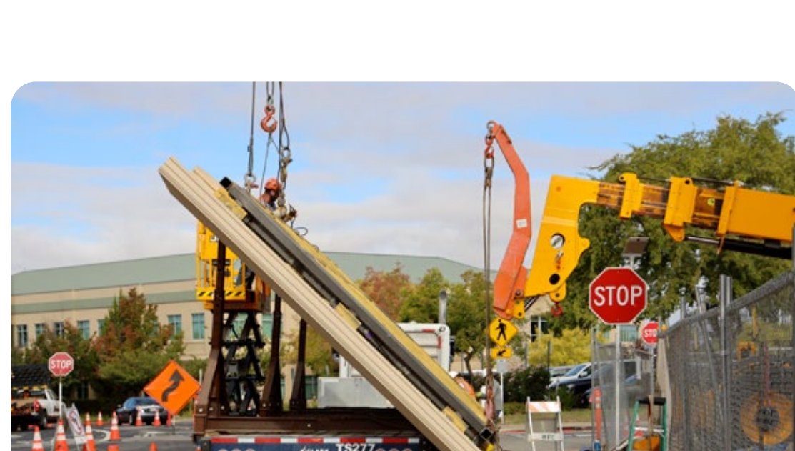
Prefabrication allows for just-in-time delivery, no lay down area is required.
