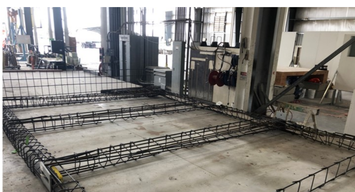
A panel in production - rebar cage for Mission Rock G
